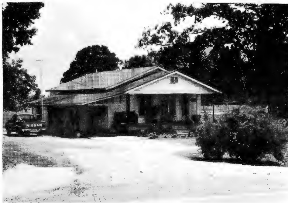
Parsonage During 1988 Renovation
